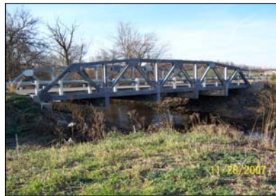
Bridge 173-0.12 over the Mad River
